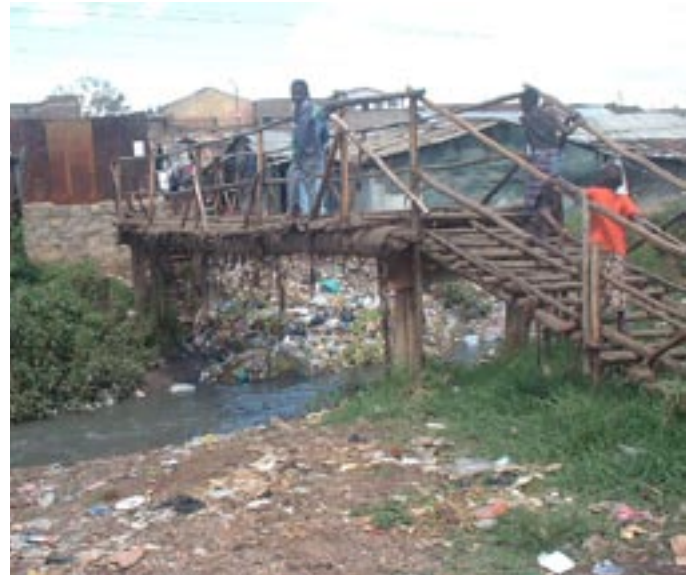
A bridge in Mukuru, a slum in Nairobi, the capital of Kenya.
